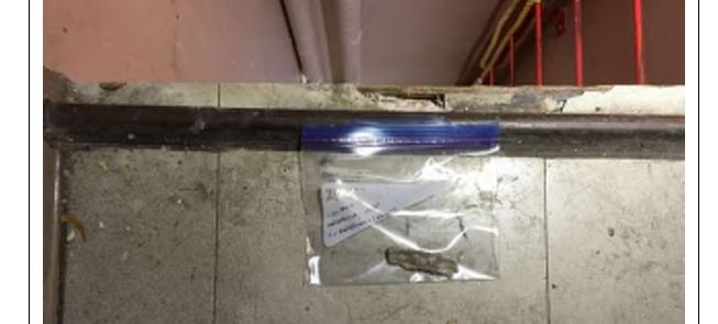
Picture No. 10: Non asbestos leveling compound beneath floor tiles (O1)
