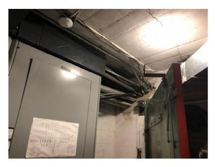
Typical Wiring without Fire Stopping
