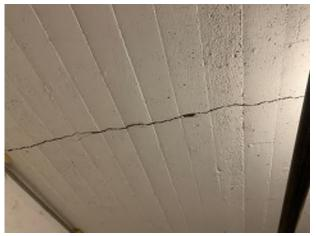
Photo #7 - Observed Suspended Slab Crack
