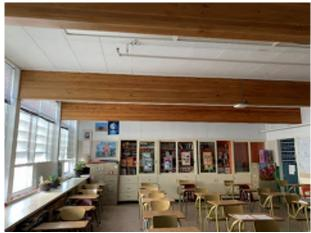
Photo #2 - Typical Glulam Roof Beams
