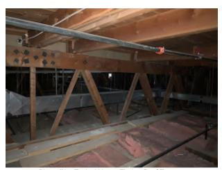
Photo #1 – Typical Heavy Timber Roof Trusses
