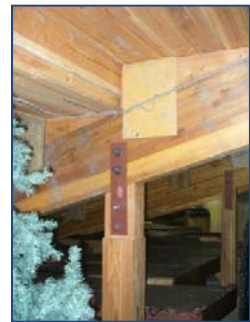
Photo no. 1 – Framing for stepped seating.
