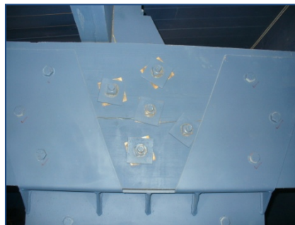
Photo no. 8 – Truss panel point connection bolts had been retightened.
