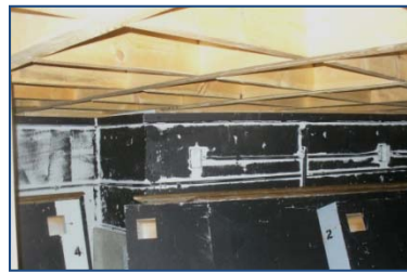
Photo no. 2 – Floor framing for the in-filled musician pit.
