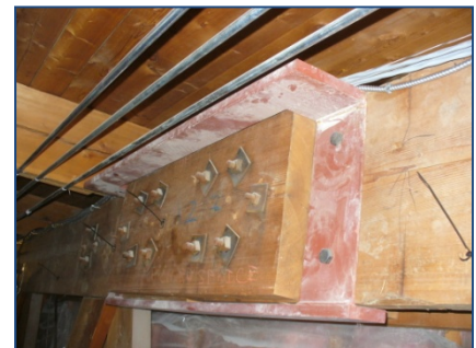
Photo no. 9 – Remedial work in strengthening truss top chord connections.
