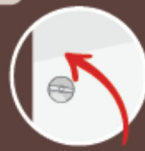
Toilet stall: area around locking mechanisms
