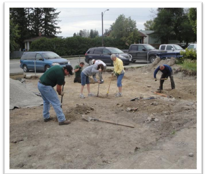
Digging Pile holes
