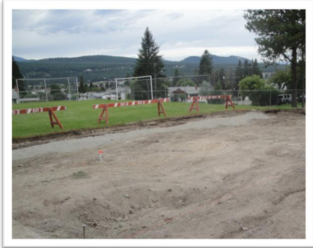
Level site with temporary fencing
