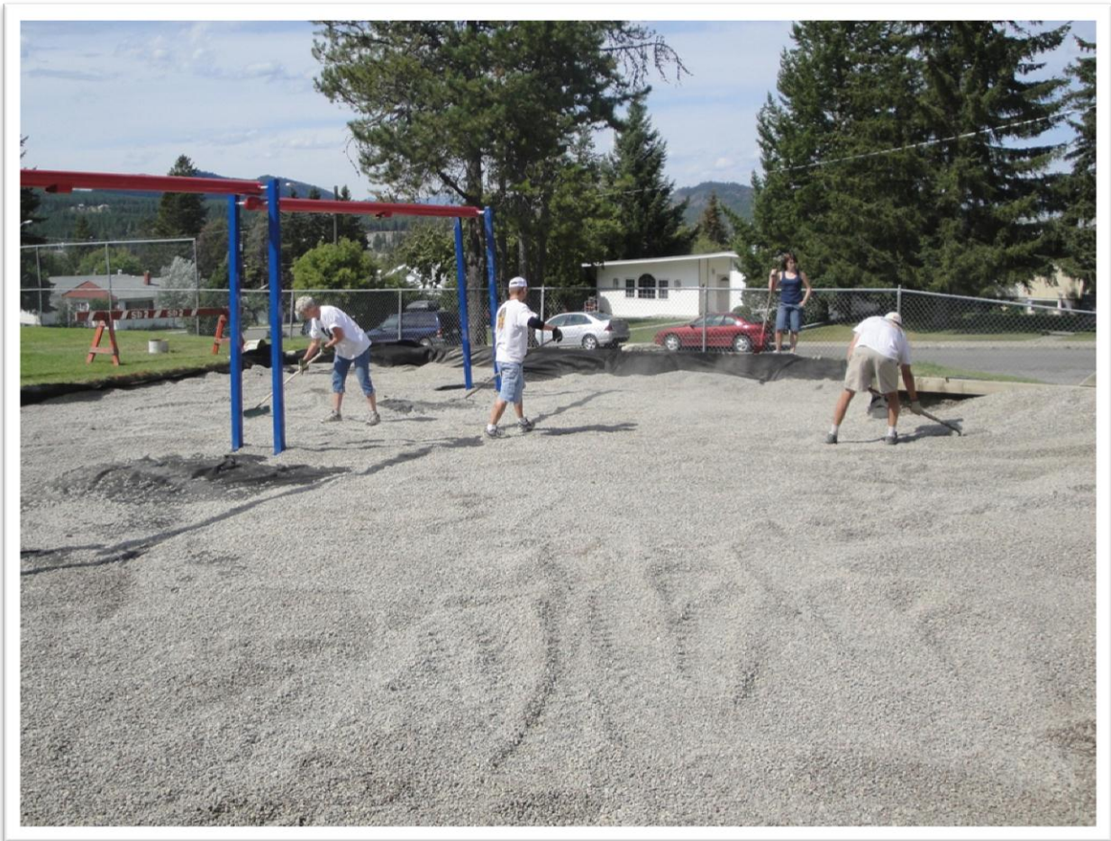
Spreading pea gravel
